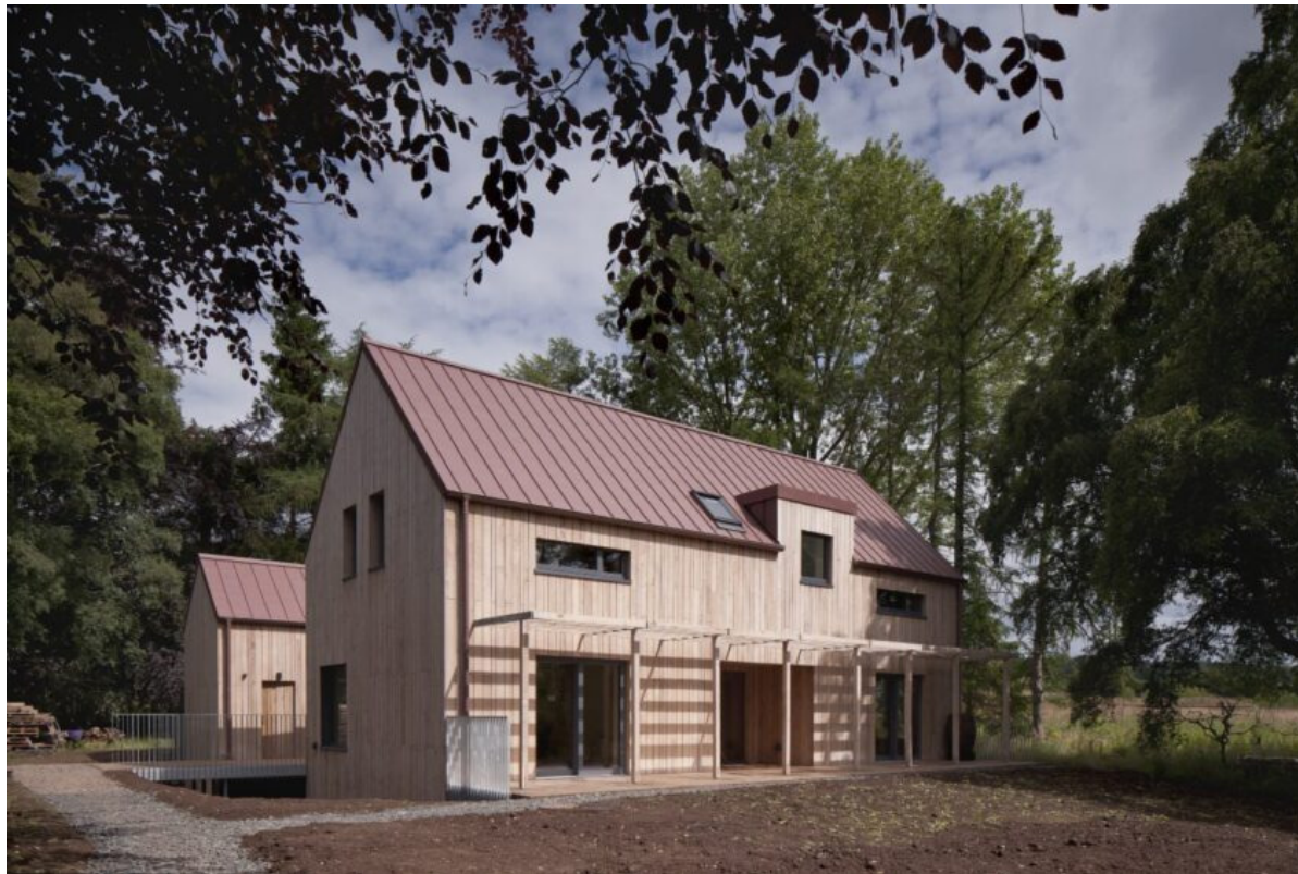
A striking Passivhaus with innovative co-living. Image: David Barbour.
