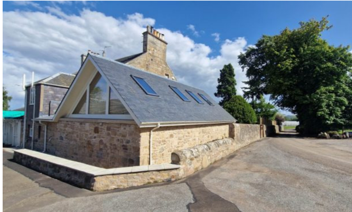
This extension was built using stone gathered from the surrounding fields. Image: DIA.
