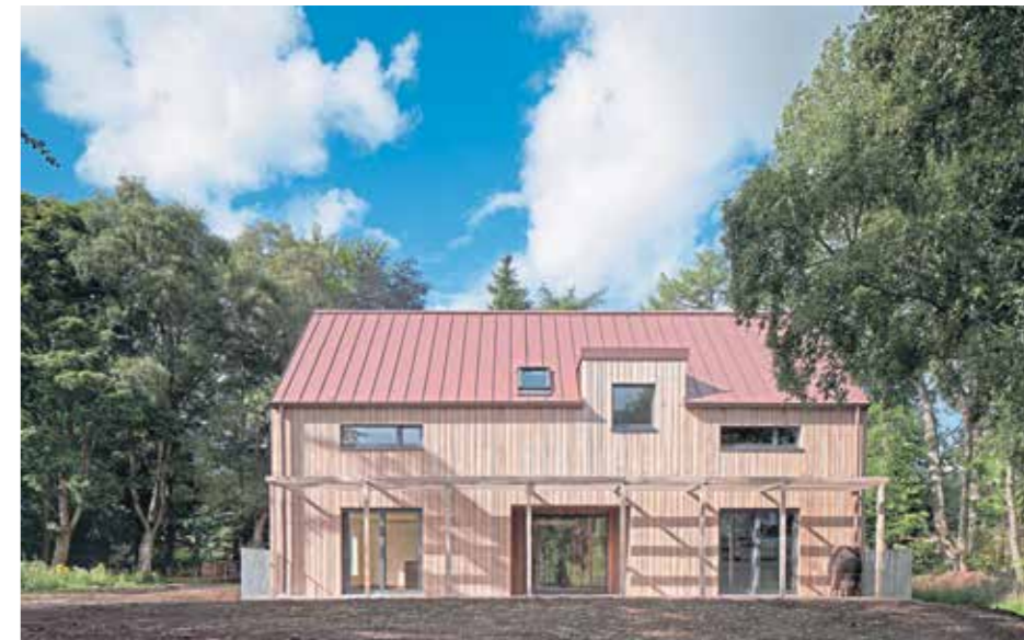
AWARD-WINNING: The Seed is set in an acre of land filled with mature trees. It is a Passivhaus, designed to be airtight through having very high levels of insulation. It was built for two households to enjoy both private and communal living.
