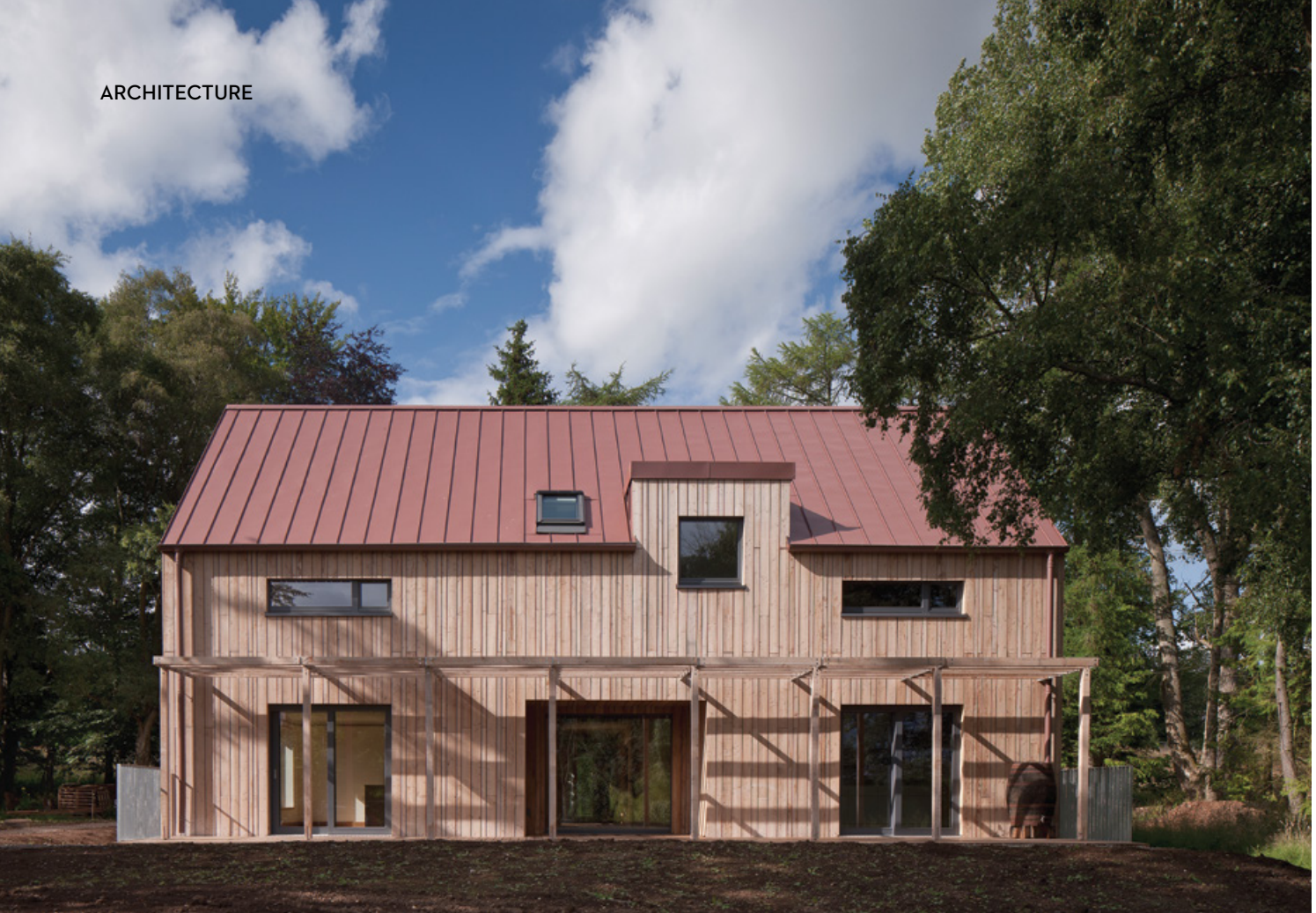
Above The south elevation has a pergola for solar shading. It forms a framework where plants can grow up and around to create a garden feature. The structural engineer on the project was David Narro Associates and the quantity surveyor was Ralph Ogg Associates. Max Fordham was the services consultant. Below One corner of the ground floor is devoted to a sauna, which is shared between the two households
