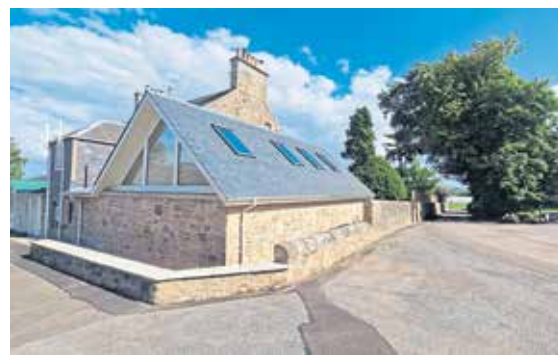
The Flaxmill at Kingsbarns was commended.
