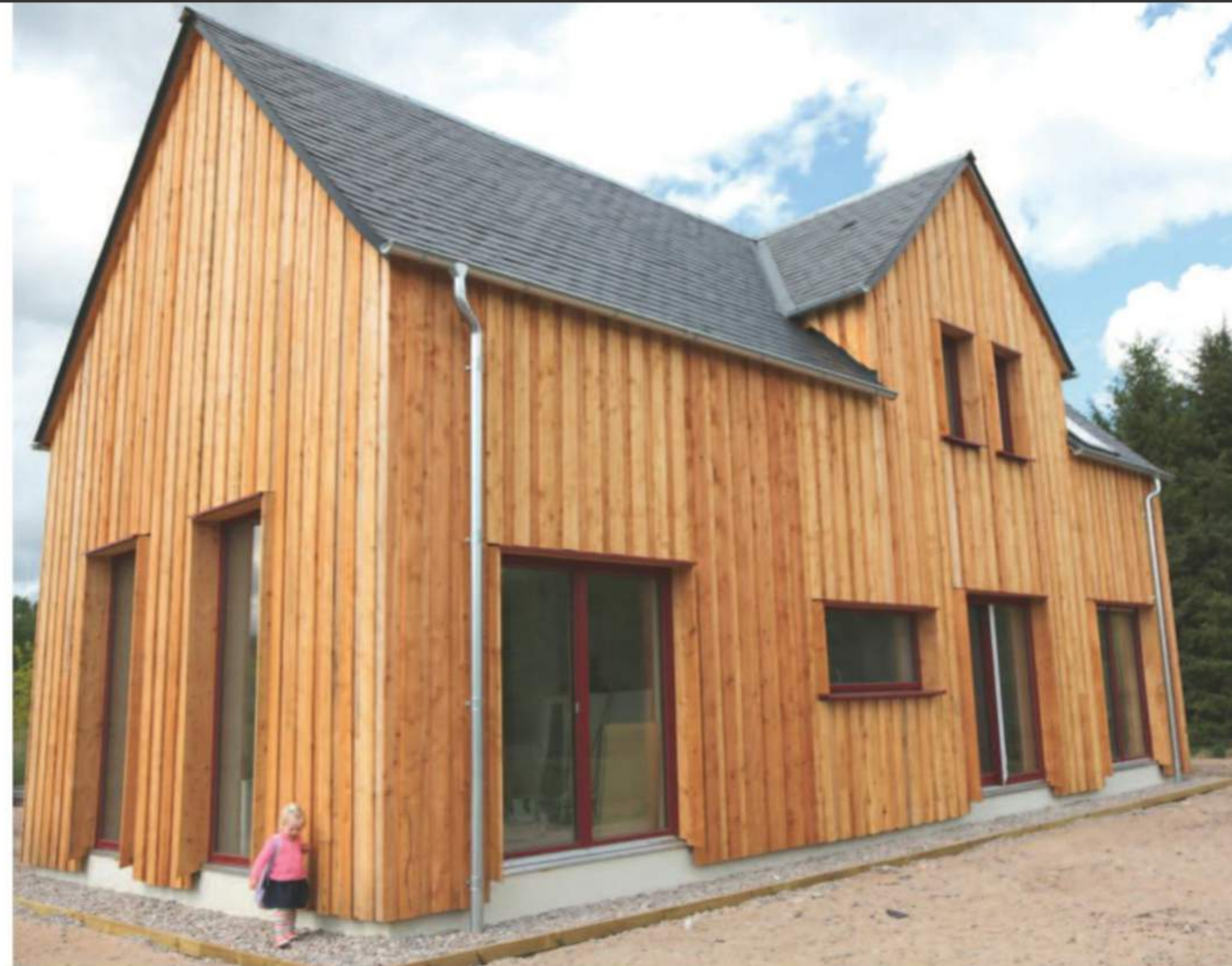
John Pullen's new family home is clad in timber felled and milled close to the site. It is heavily insulated (right) - and the thermal image testifies to its heat efficiency.
